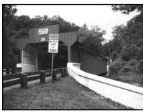
Geiger's Covered Bridge located near the village of Weidasville spans the Jordan Creek. The structure was built in 1858, has stone abuts and a double wooden floor. Geiger's is 120 feet long with a water pipe running through it from which water was pumped from the Jordan Creek to a nearby farm. The County of Lehigh maintains this bridge.
